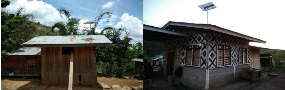
Diagram 7: Roof-through Pole mounted installations on GI roofs
