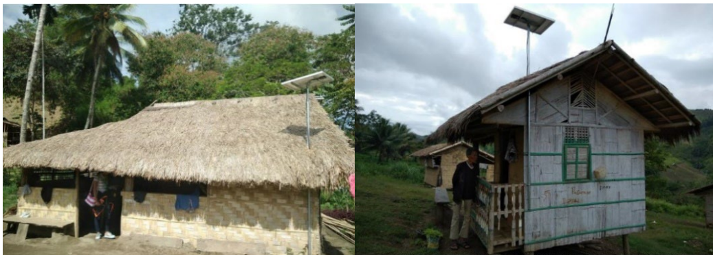
Diagram 8: Roof-through Pole mounted installations on thatched roof
