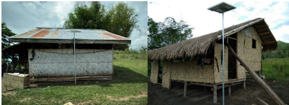
Sample Roof-side Pole mounted installation
